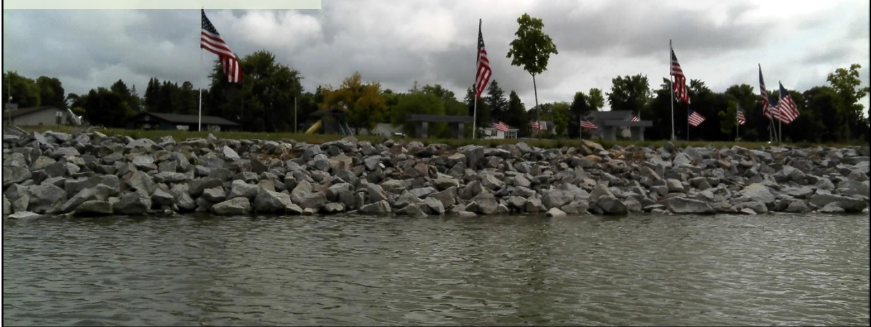
Erosion along south shore
